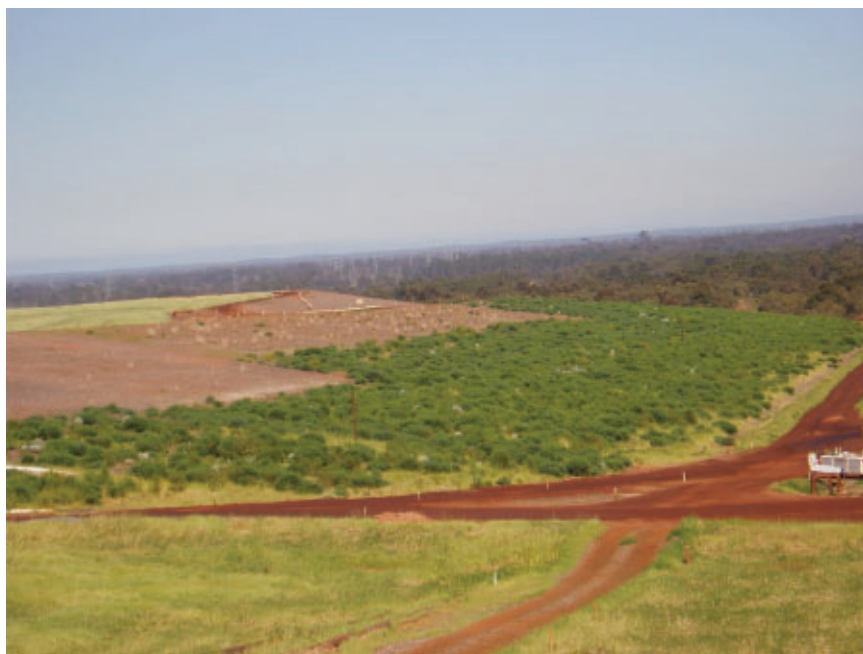
Fig. 5. Examples of surface covers in bauxite residue progressive closure: wood mulch, rehabilitation and pasture.
