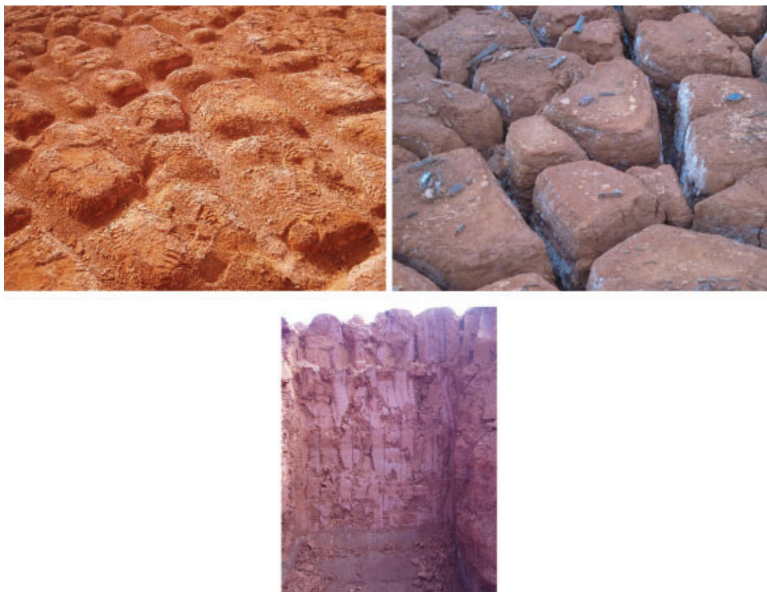
Fig. 3. Surface cracking of residue mud as it progressively dries, with evidence of cracking within the profile.
