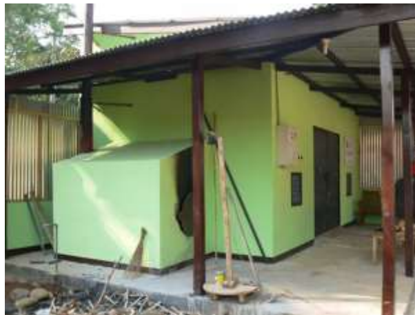
Figure 5. The completed drying chamber.
