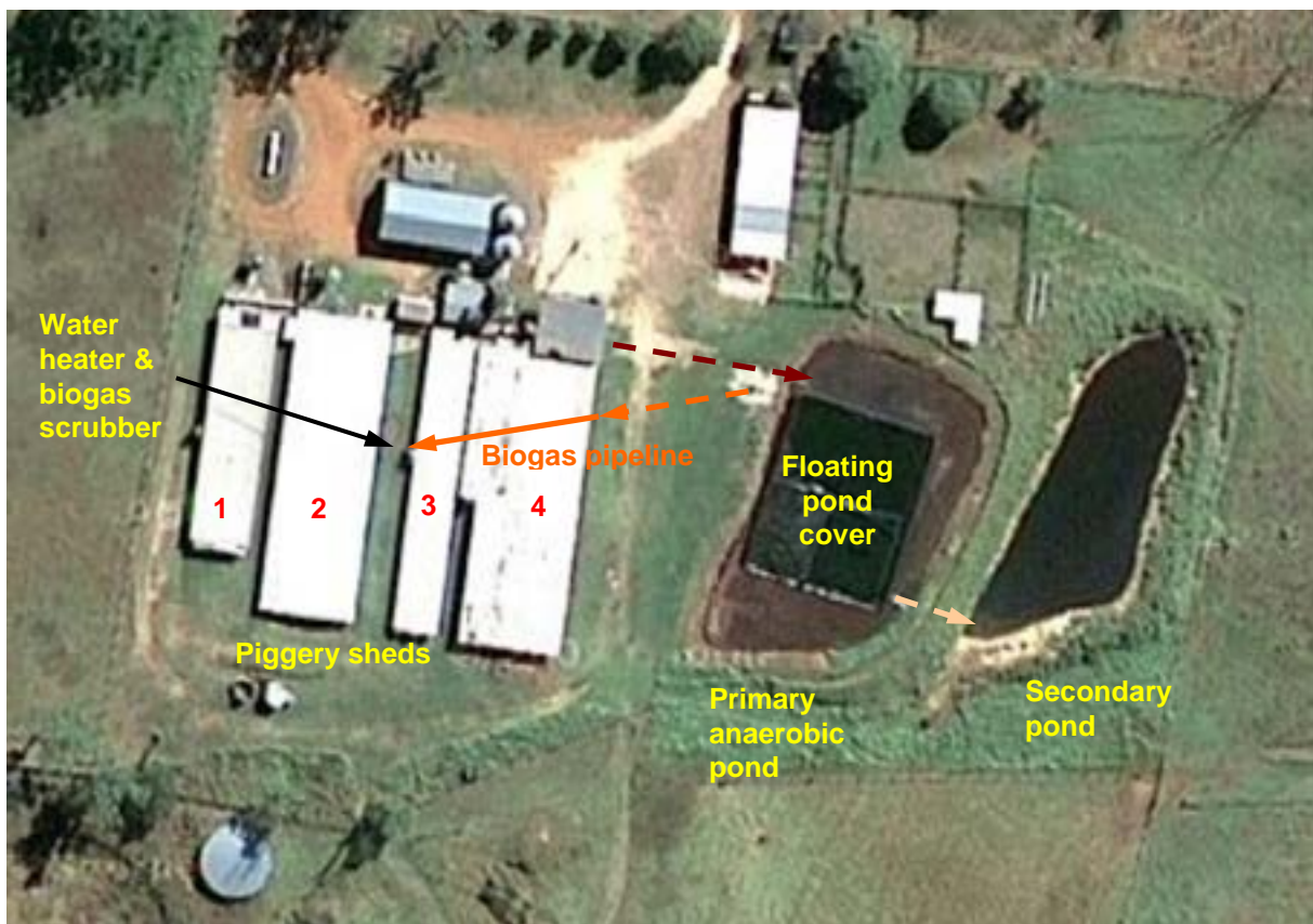
Figure 2. Aerial photograph of the piggery showing the locations of the partially covered primary effluent pond, biogas pipeline, water heating unit and biogas scrubber.
