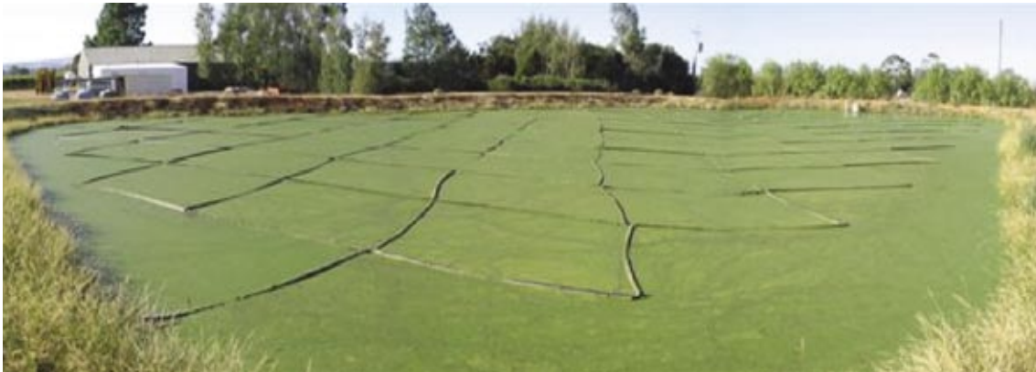
Photo 3. Ventura Vineyard irrigation lagoon, Adelaide. The objective of DWT on this lagoon is to maintain very low levels of suspended solids for the drip irrigation system and to minimise evaporation ( photo courtesy Robert Bell ).
