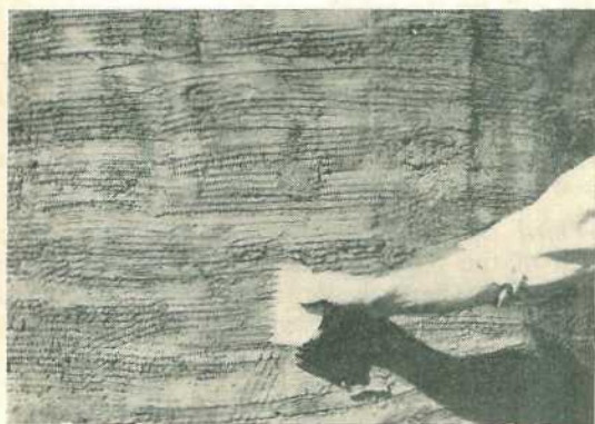
Plate 6 Roughened Second Plaster Coat Ready for the Final Coat.
