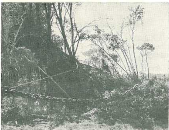
Pulling virgin scrub using a cable and chain.
