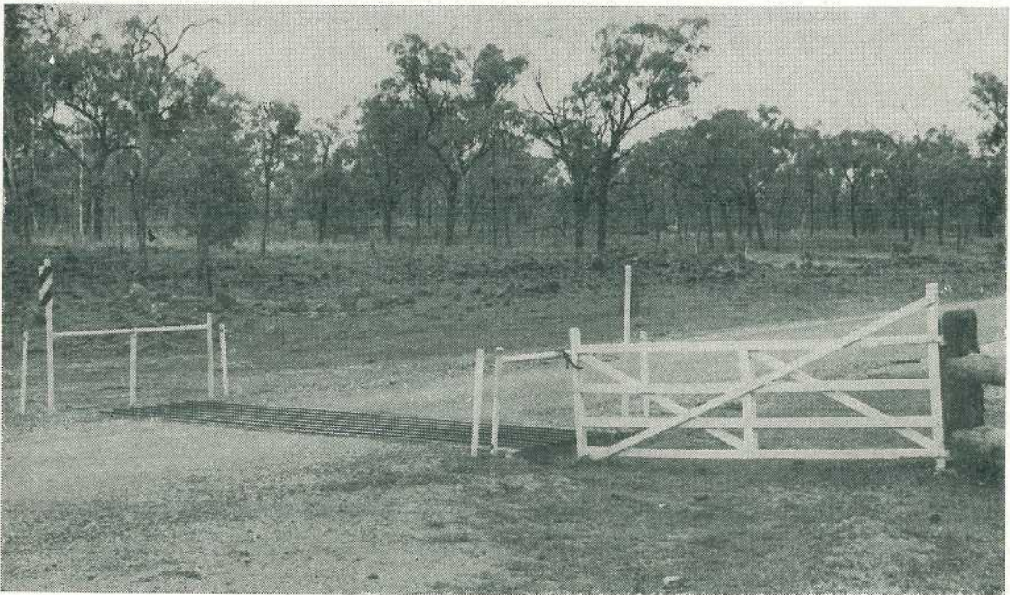
It is often necessary to have a gate close to a grid so that cattle can be put through the fence.
