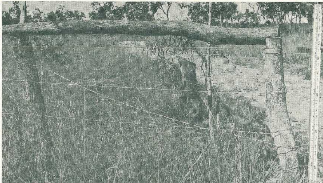
Strainer assemblies are more likely to fail if the horizontal stay is short, if the posts are set too shallow, or if the diagonal brace cannot be kept tight.
