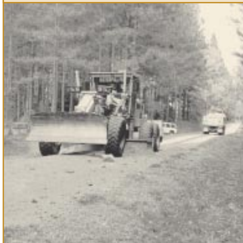
Gravelling a section of Dalrymple Road in Abergowrie State Forest (Ingham forestry district). DPI Forestry undertook a review of its road practices during 1998-99, including road construction and maintenance, to improve productivity.
