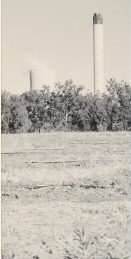
Stanwell Power Station is establishing its seed orchard on this site, providing an environmental buffer-strip, a greenhouse emission tool and seed stock for western forest plantations.
