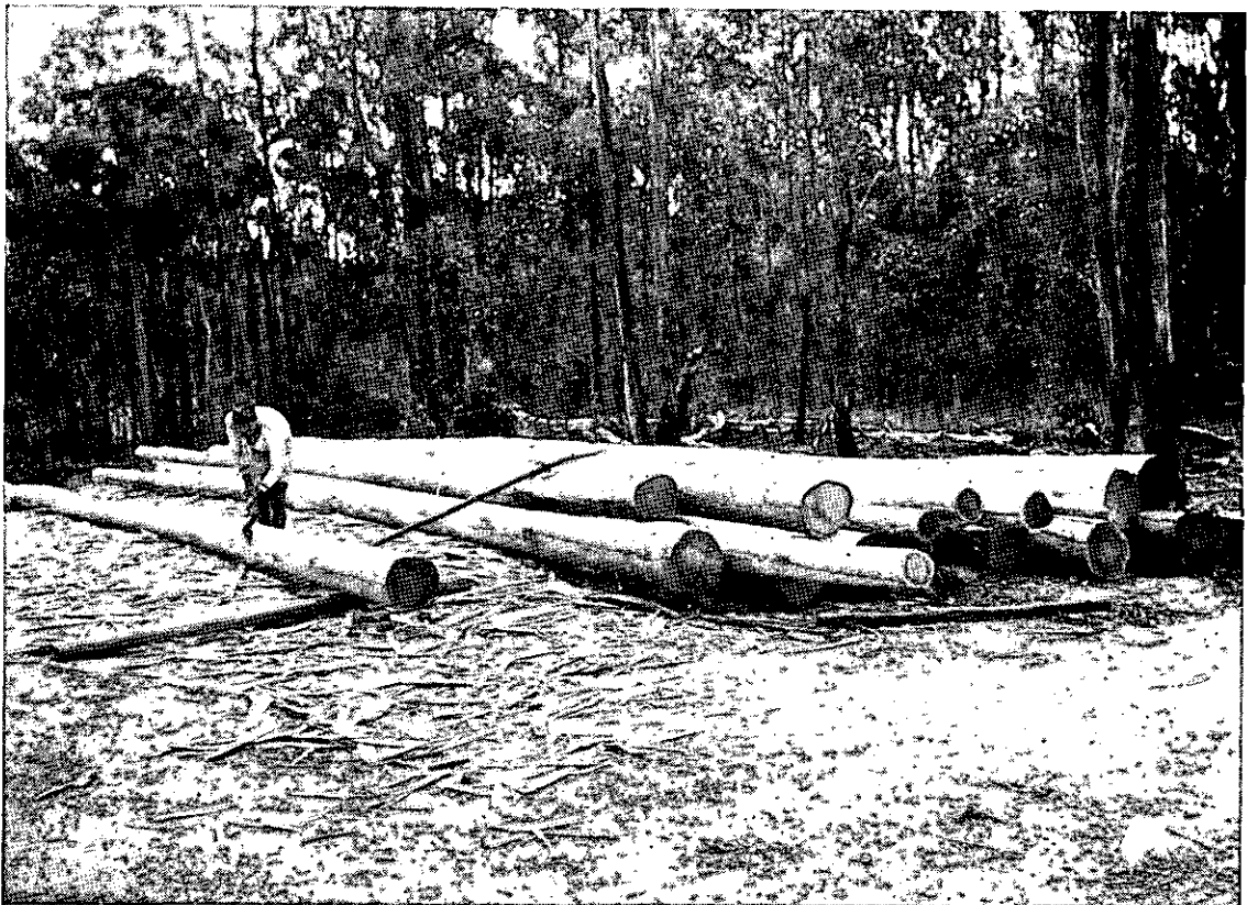
POLES FOR EXPANSION OF ELECTRICITY SUPPLY TO RURAL AREAS.
