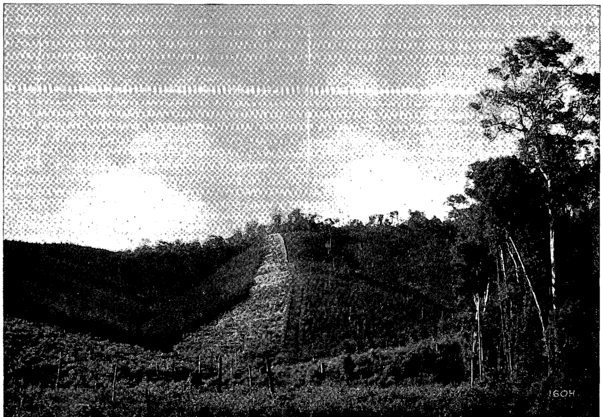
INTERNAL FIRELINE (CENTRE) AND SCRUB FIREBREAK (TO P AND RIGHT). HOOP PINE PLANTATION, MARY VALLEY DISTRICT.
