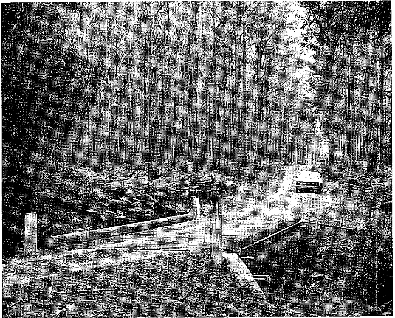
MELLUM CREEK BRIDGE—BEERWAH PLANTATION AREA—Constructed during the year at a cost of $3,970: background of Loblolly Pine aged 34 years—Compartment 7, Mellum Logging Area.
