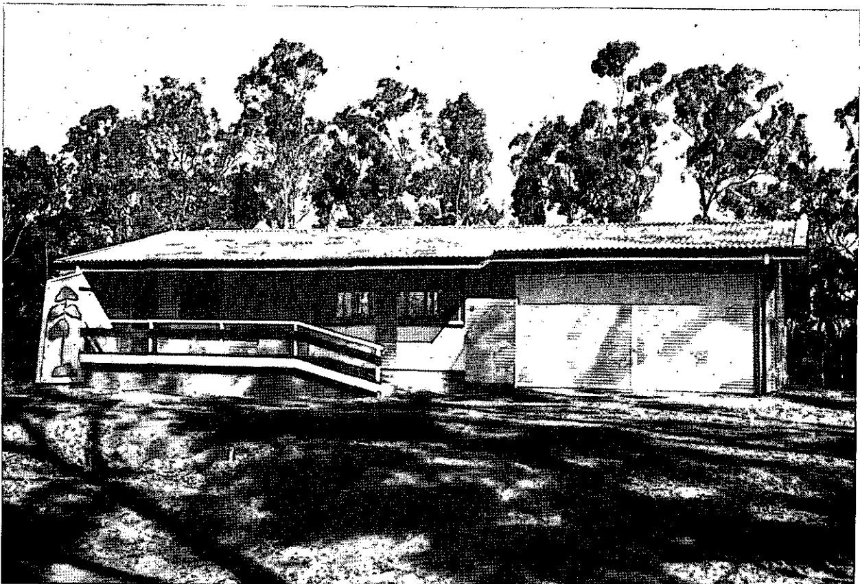
COMMUNICATIONS CENTRE—BUNYA STATE FOREST—ERECTED 1963-64 The nerve centre of radio communication for the Department
