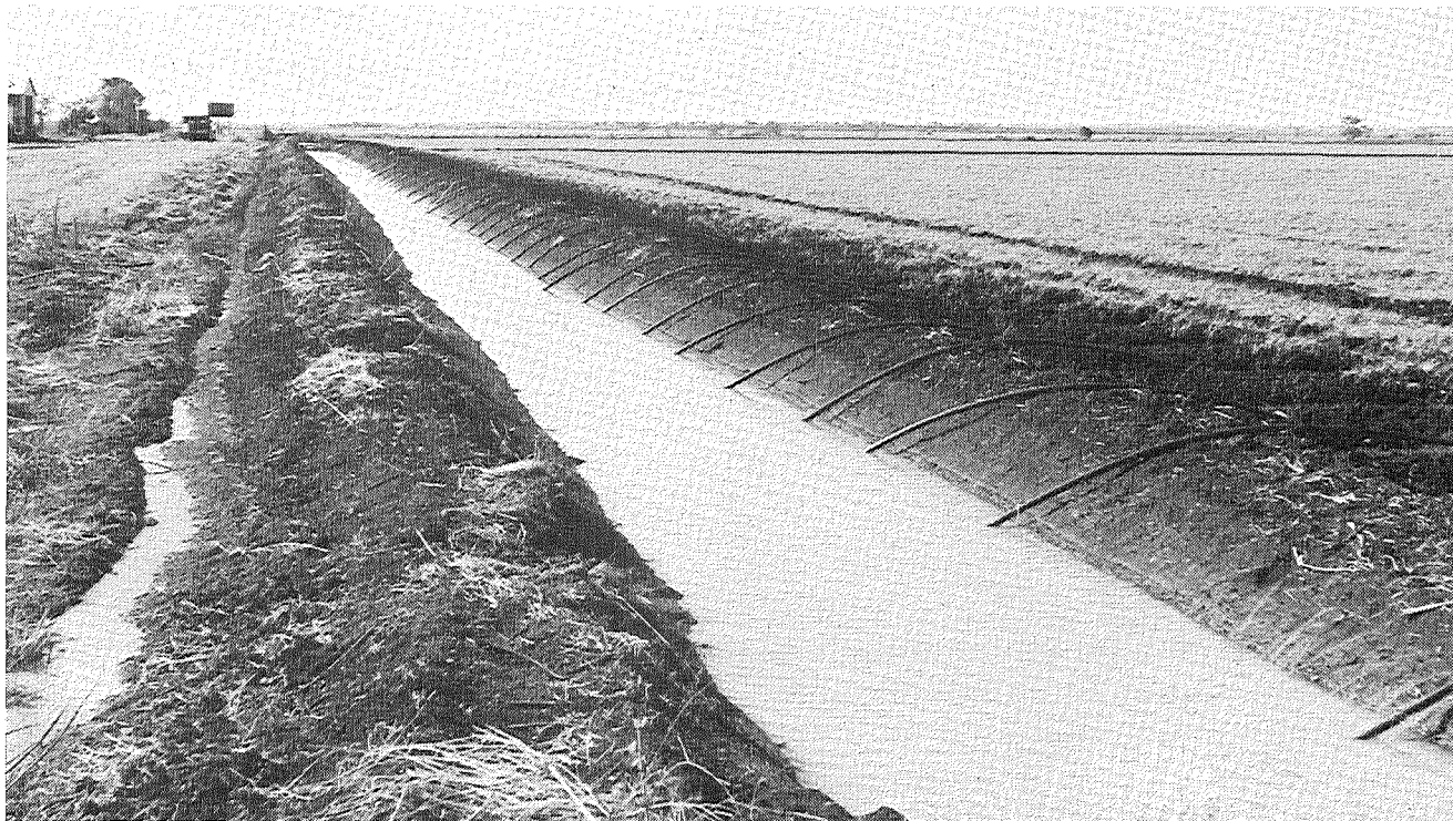
Weeds, particularly annual summer weeds, have become a problem in the Emerald Irrigation Area. Weed-free head ditches, such as the one in the picture, allow water to flow freely and permit easy use of siphons.
