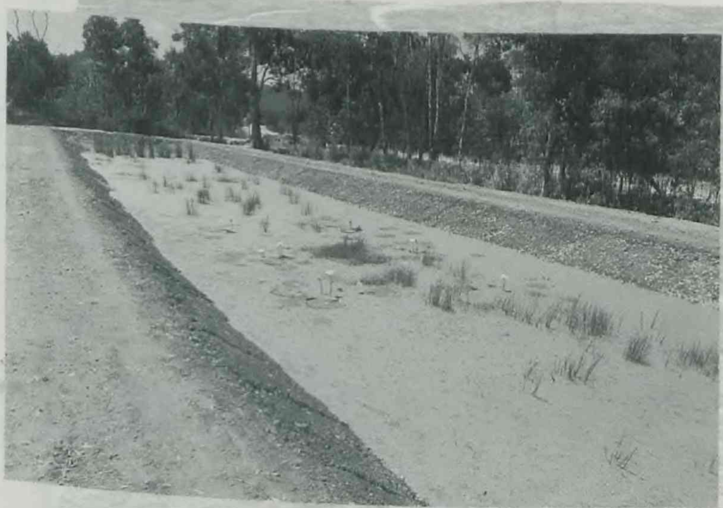
Joint Cairns City Council-DPI artificial wetland, at Edmonton south of Cairns, being used for pilot testing of wetlands for sewage effluent polishing.
