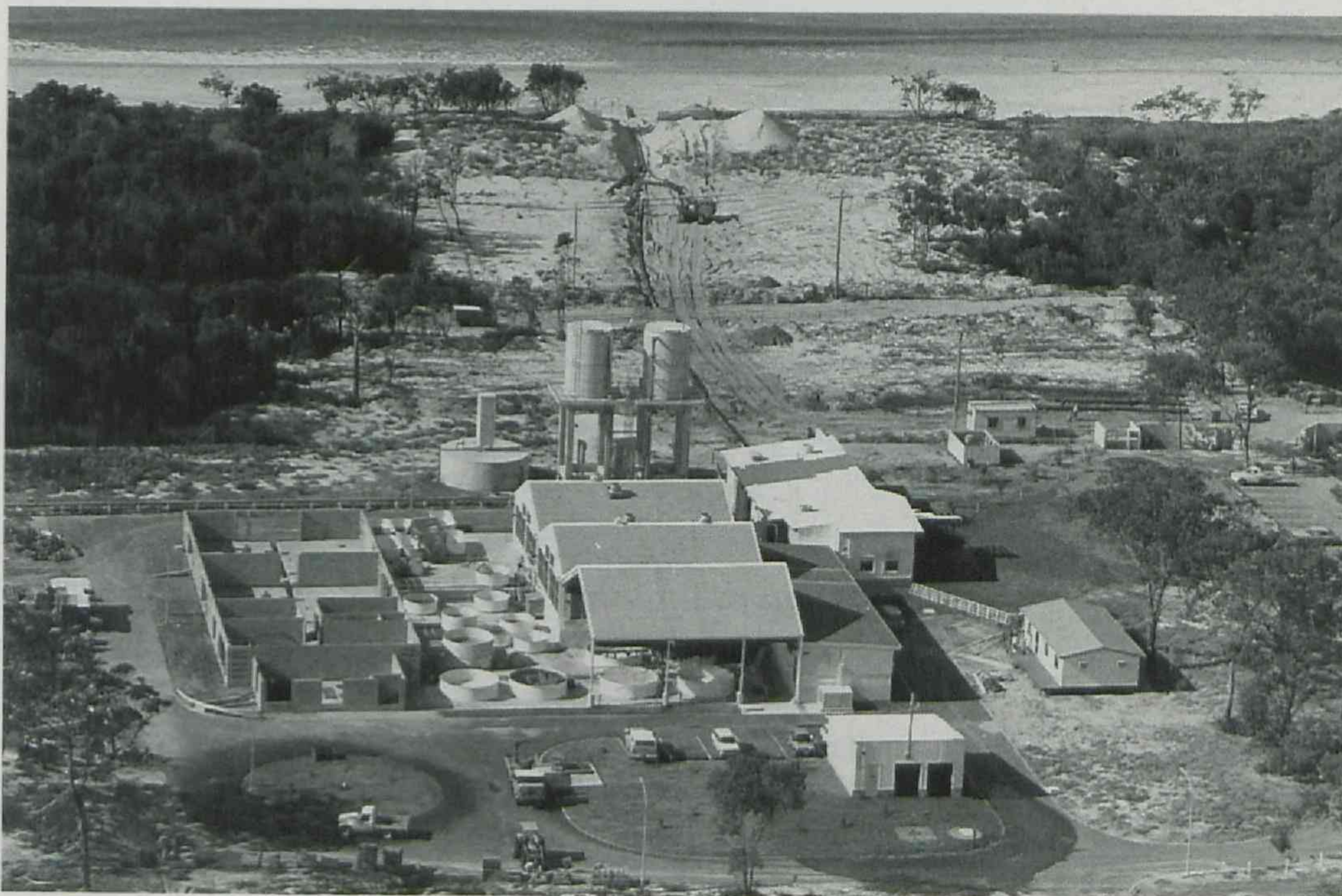
The Bribie Island Aquaculture Centre at 30 June showing the prawn nursery and algal production facilities, and the header tanks for salt and freshwater supplies (centre); the seawater pipeline (top centre); and the prawn maturation building under construction (left centre).
