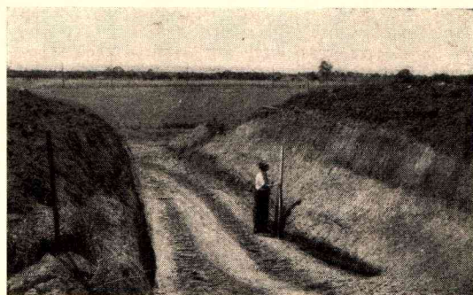
Plate 6.—A Silage Trench With Adequate Wall Slope to Ensure Tight Packing of Silage Against the Sides.
