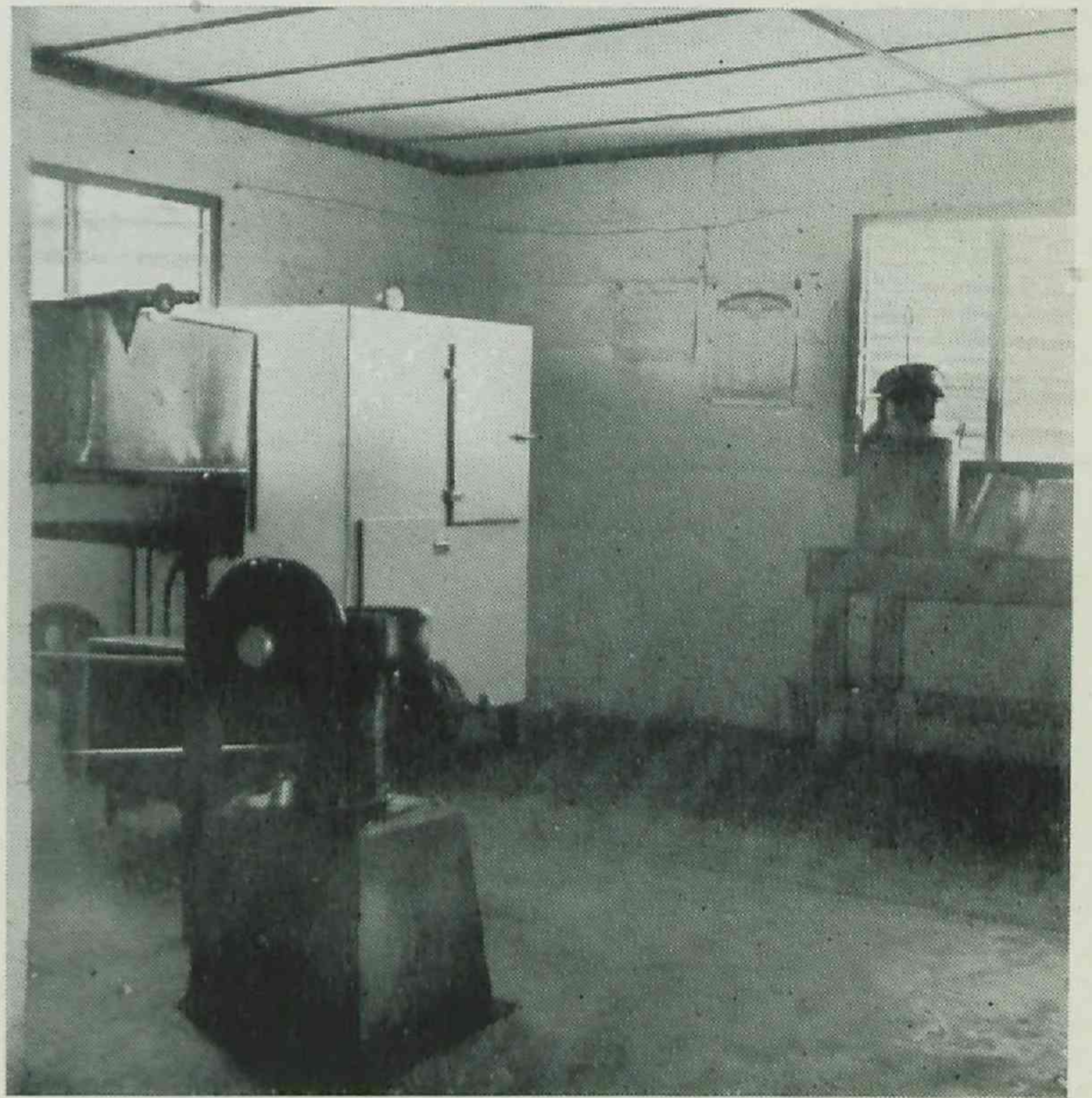
Plate 15. The Separator Room at a Modern Dairy Shed.
