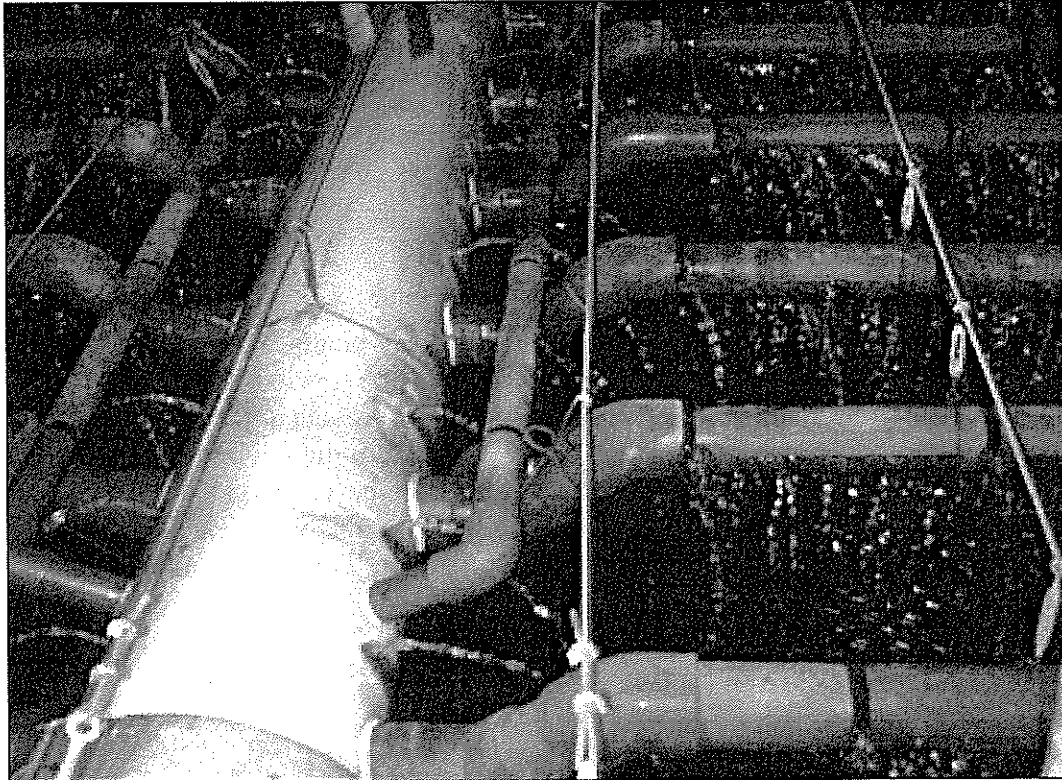
Figure 9 Trickle filter system for Roi fish farm
