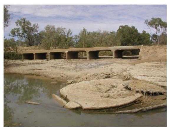
**Plate 13** Punchbowl crossing on the Flinders River has good-sized culverts that would not restrict fish passage.
