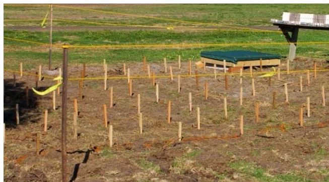
Figure 7 Stakes installed at Dalby
