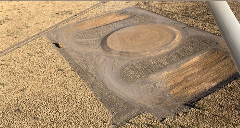
Photo 4. Completed Flood Refuge Mound. Photograph courtesy of A.A. Company Pty Ltd.
