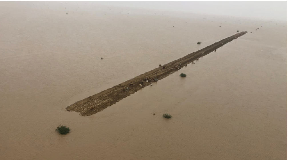
Photo 1. Livestock on a purpose-built bank (effectively an elongated rectangular flood refuge mound) during the 2019 Monsoonal Flood. High volumes of soil per animal area are required with this design. Square or circular FRMs are therefore more efficient per head. Photograph courtesy of A.A. Company Pty Ltd.
