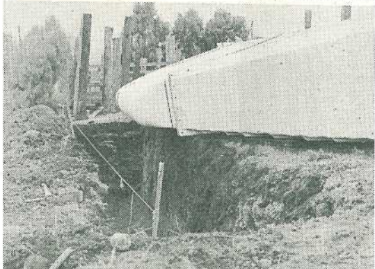
The fibreglass dipping vat is ready for lowering into the hole.
