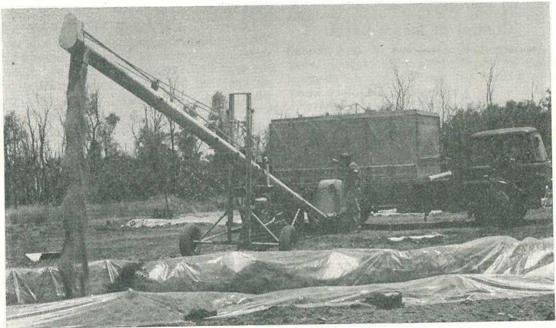
Filling an underground pit by augering direct from a field bin.
