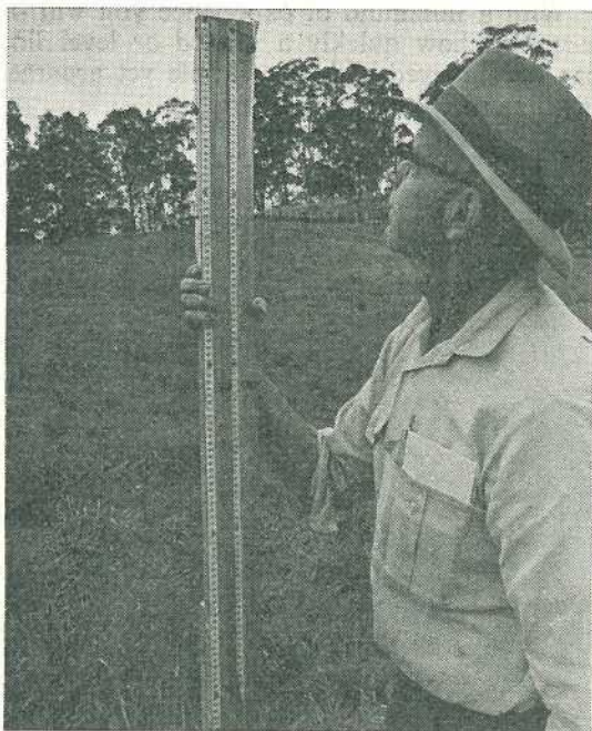
Holding the staffs together to check water height. If the tops of water column don't agree there could be a bubble in the hose.
