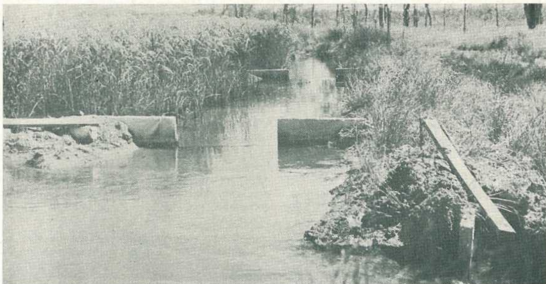
Bay to bay flood irrigation with concrete checks. Water is being drained from this crop.
