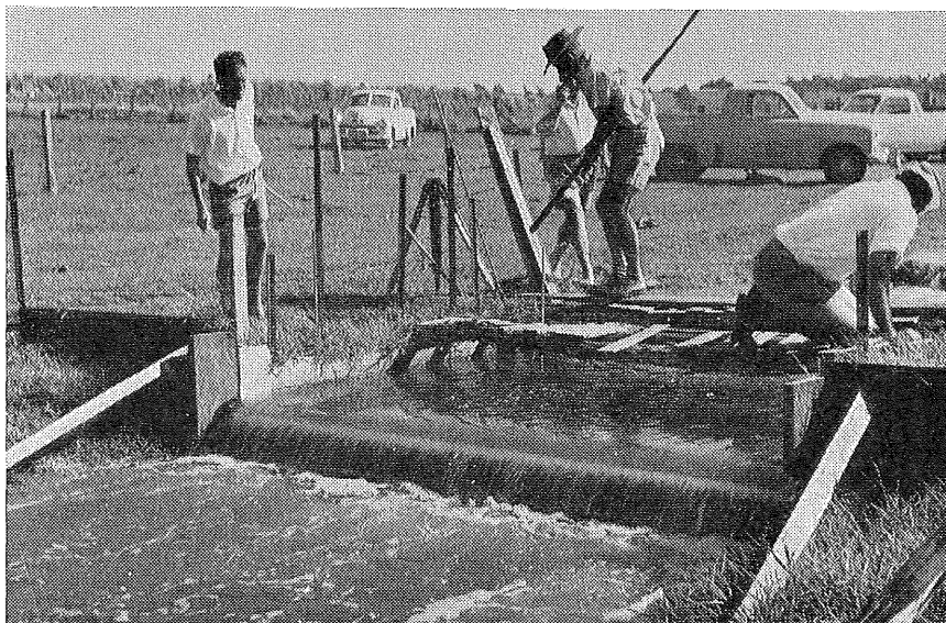
Fig. 2.—Measuring weir. Measurement of head of water flowing over the weir is being made from a piano wire stretched across the approach channel 6 ft above the weir.
