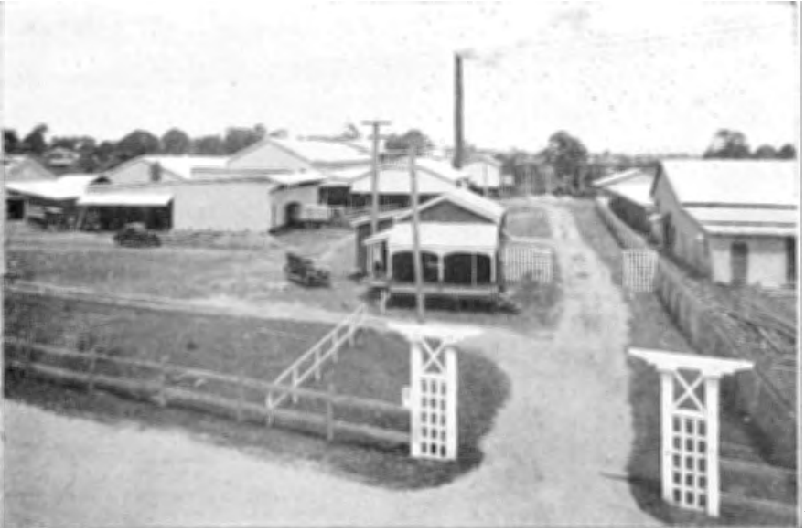
General View of a Brisbane Plywood Factory.
