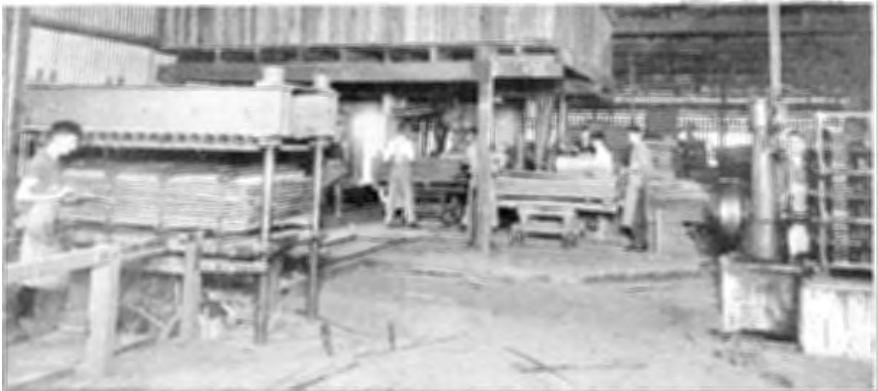
The Glueing-Process. Glue-spreader and Hydraulic Press in Operation.
