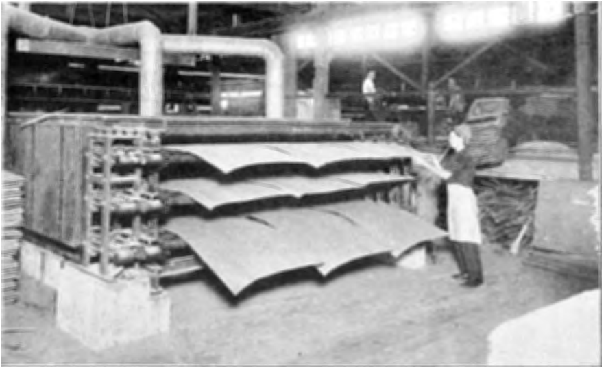
Drying Veneers in Steam-heated Kiln.
