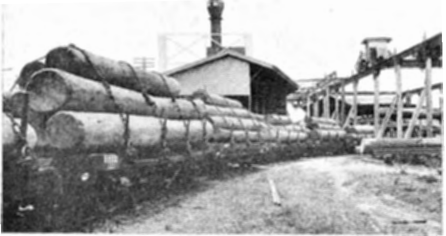
Hoop Pine Logs at Plywood Factory.
