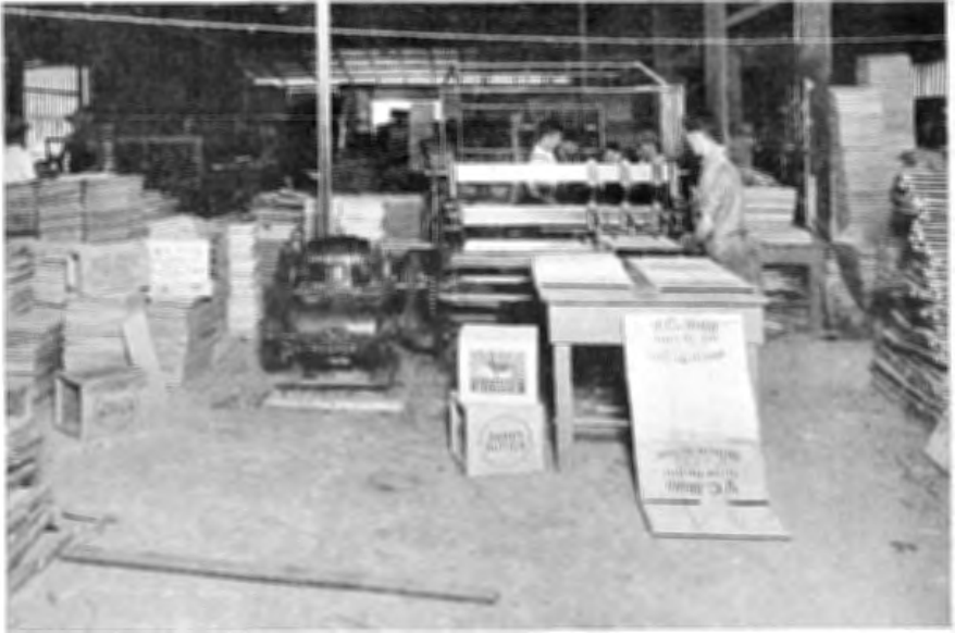
Manufacturing Boxes from Hoop Pine Veneer in a Brisbane Factory.
