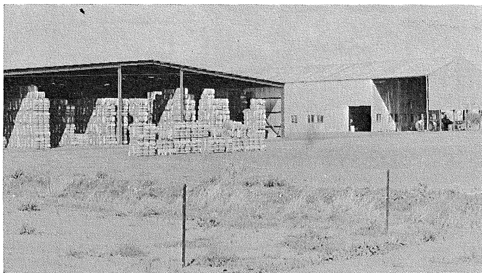
Because of the successful production of irrigated cotton at St. George, a cotton gin has been located in the area.
