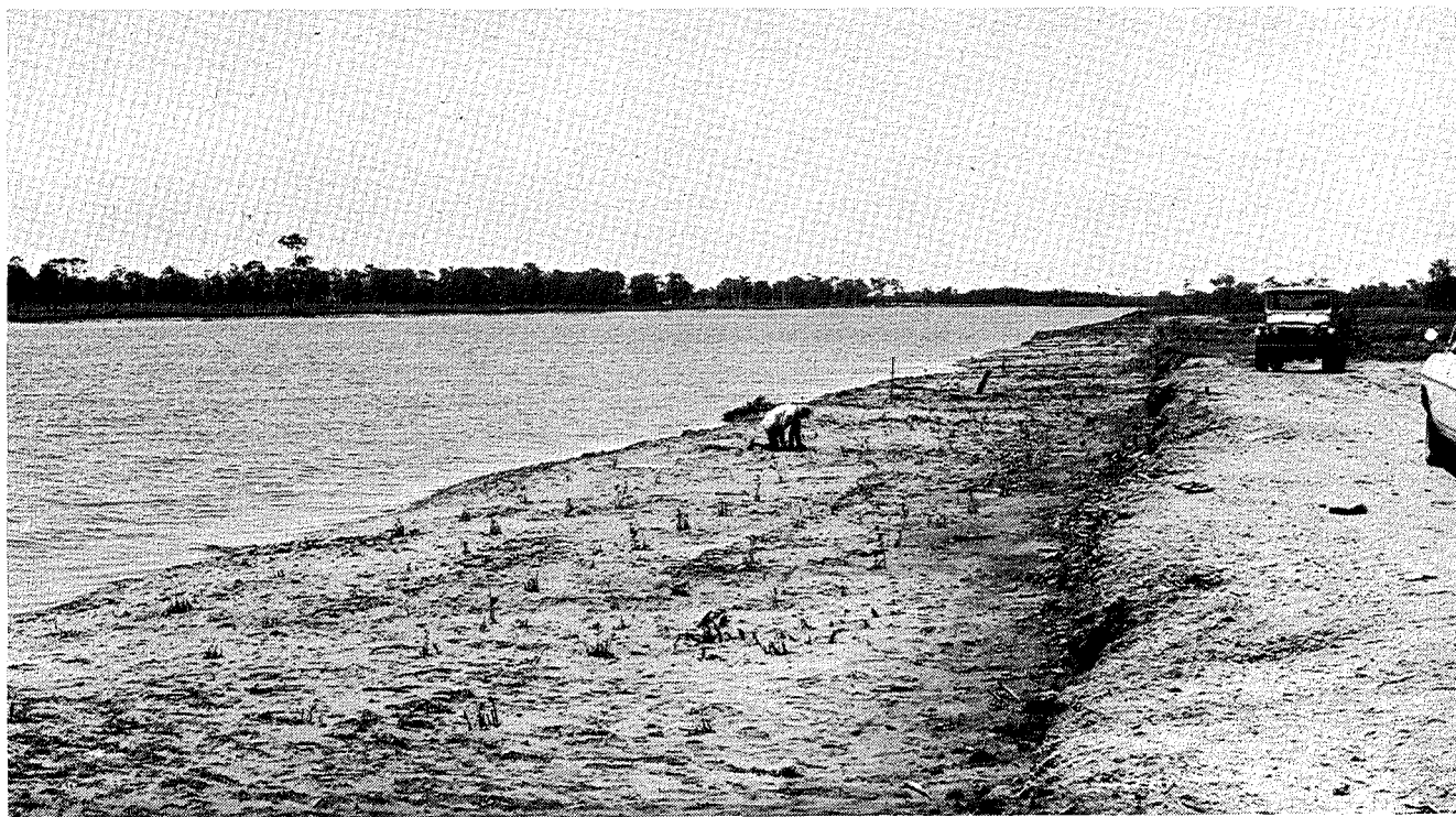
Establishment of mangroves to stabilize the drainage canal at the new Brisbane International Airport.
