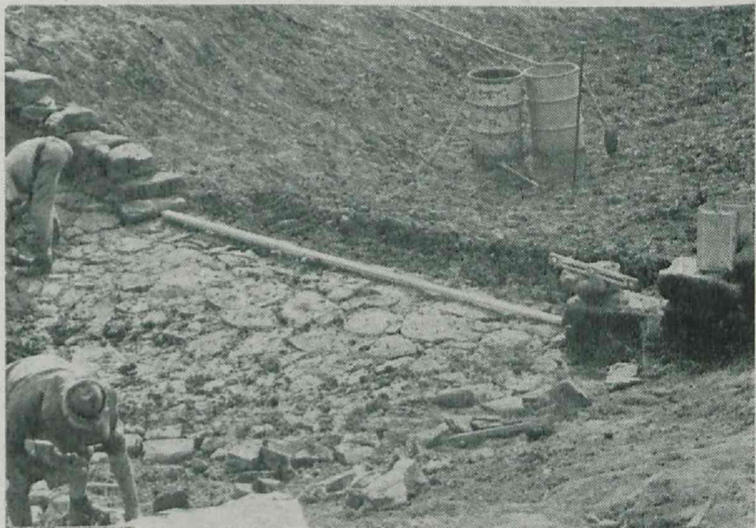
Gully control measures such as this sill construction (above and below) now constitute a large proportion of extension activities by Soil Conservation Branch officers in the Miles district.
