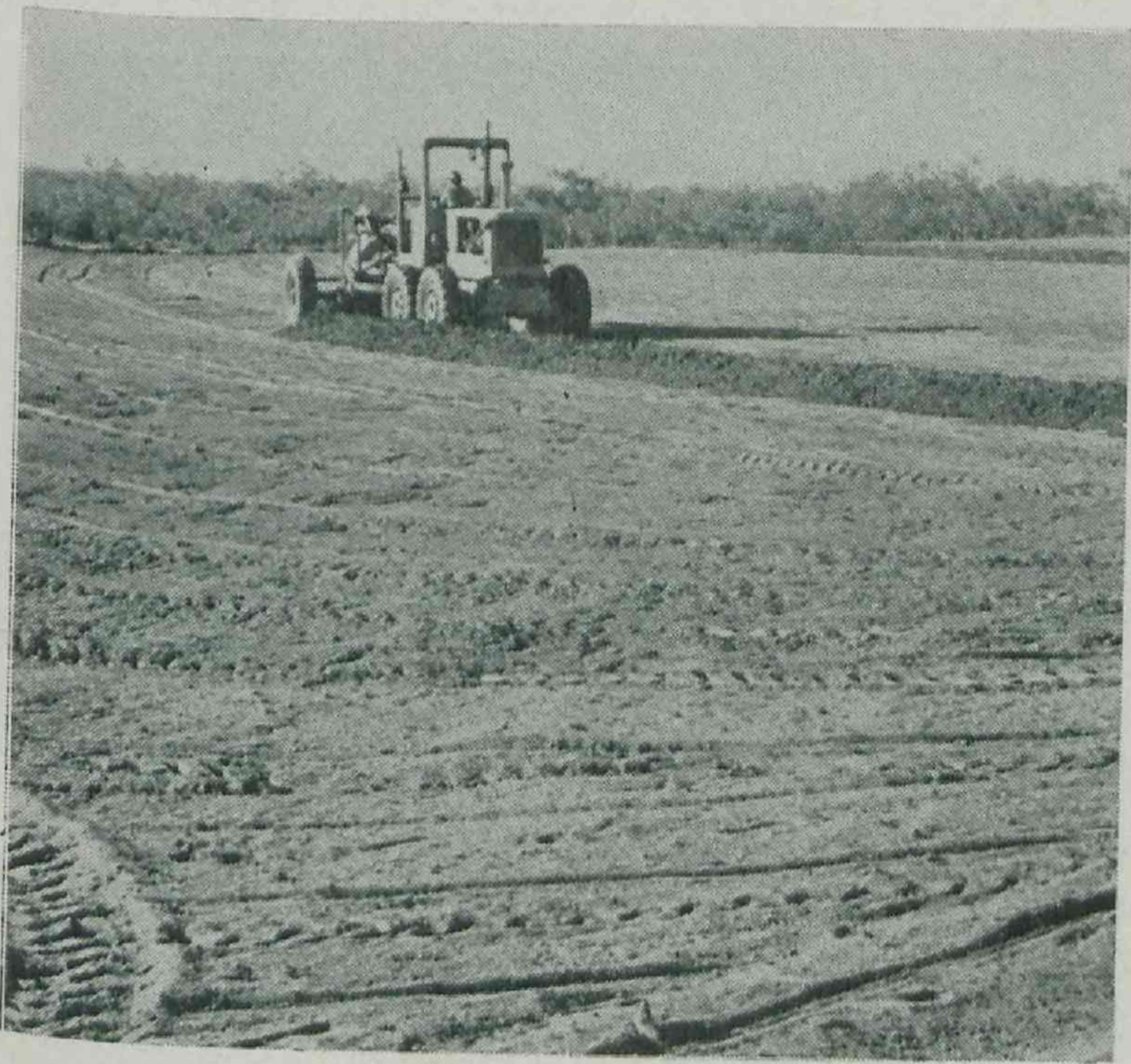
A power grader constructing parallel contour banks in the Mareeba District.
