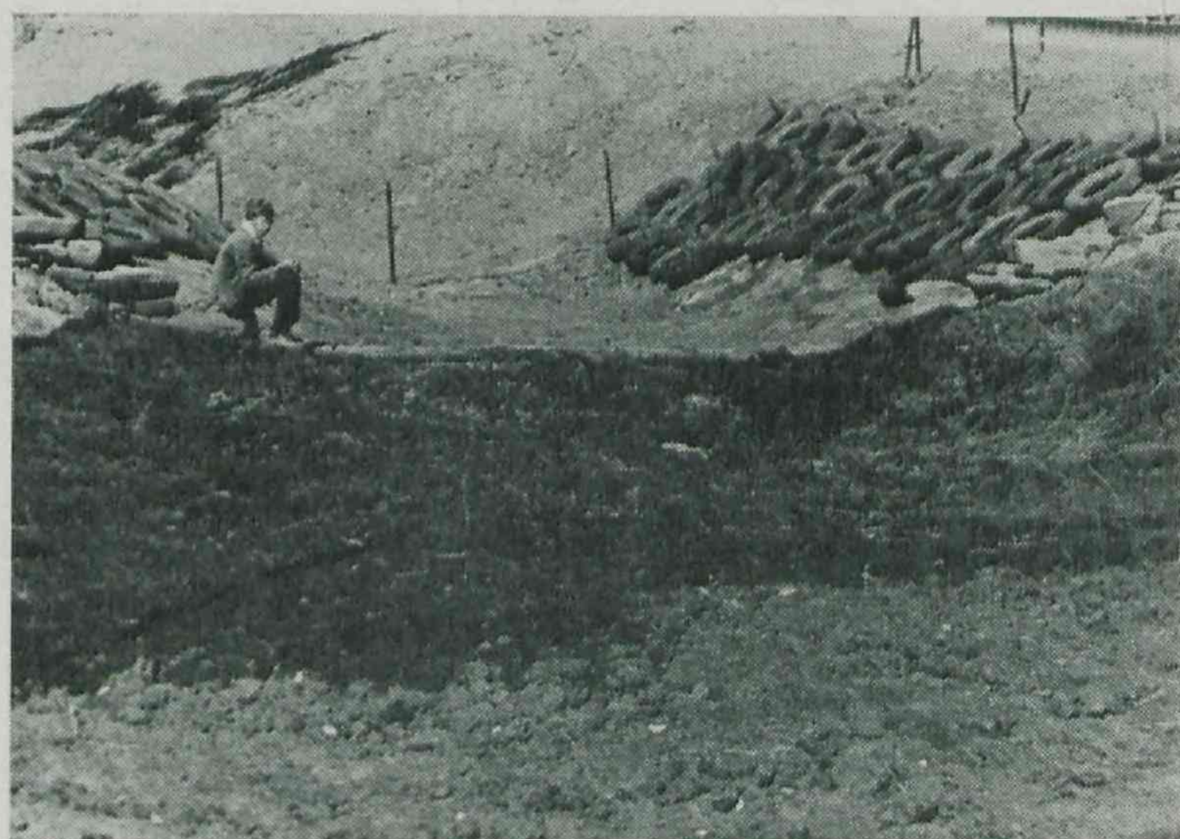
Gully control measures such as this sill construction (above and below) now constitute a large proportion of extension activities by Soil Conservation Branch officers in the Miles district.
