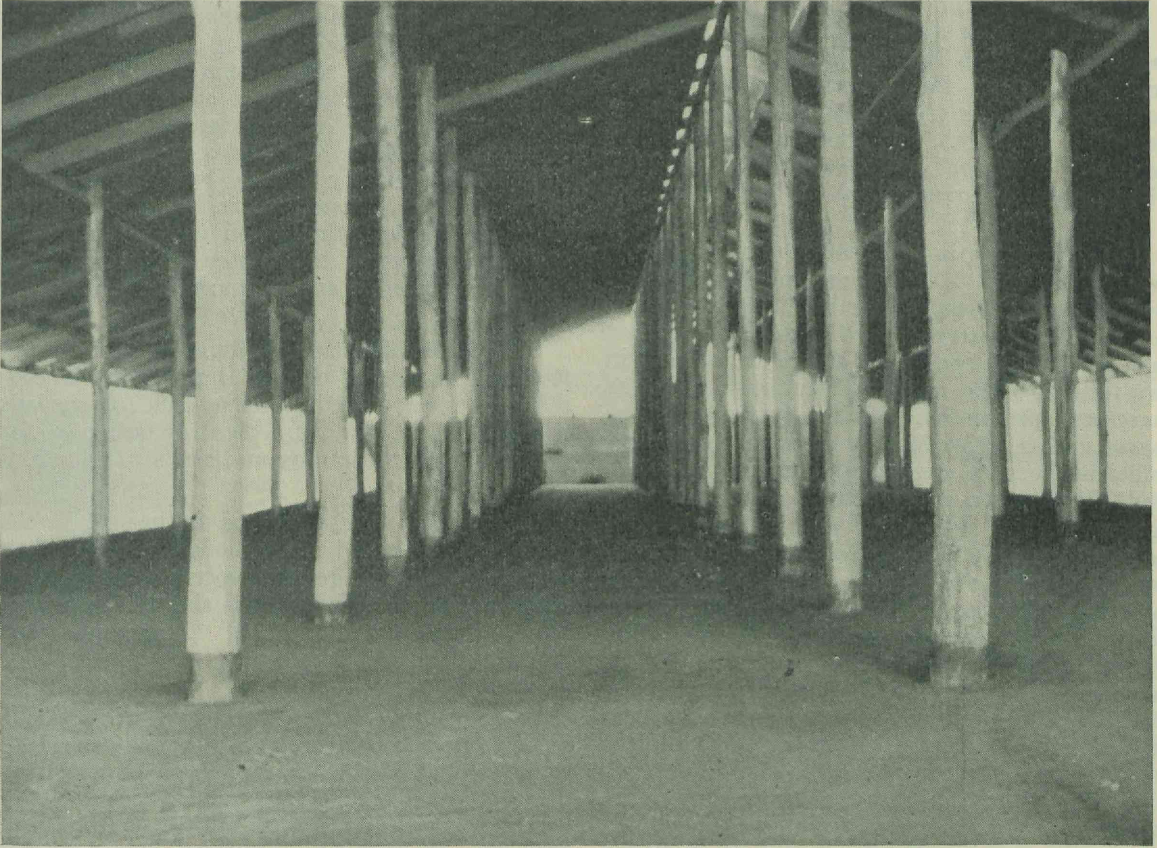
Plate 3.—Interior of Bulkhead Store. The centre poles are 17 ft. high; the floor is lined with bitumenous sheeting.
