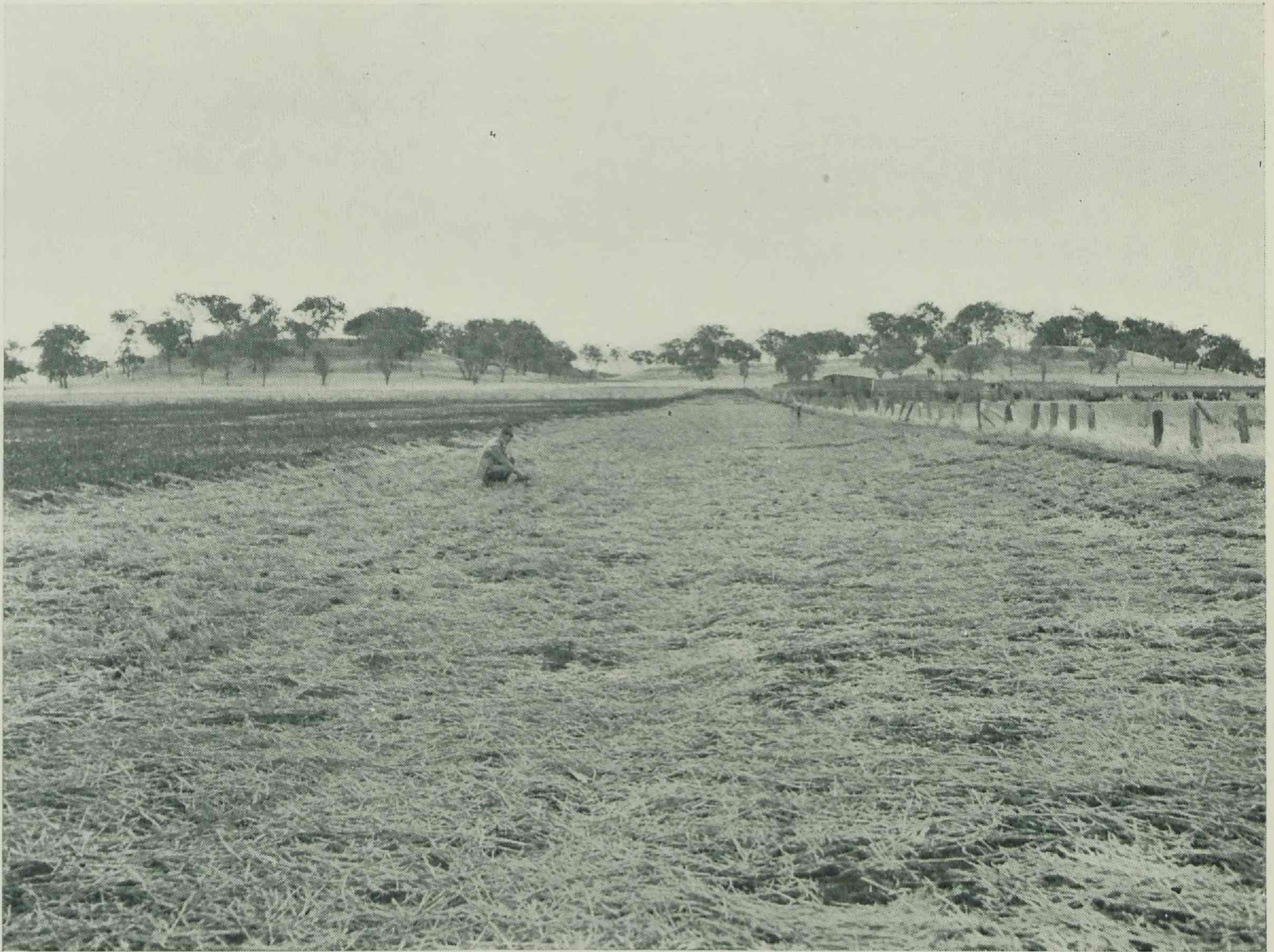
Plate 1.—A prepared waterway on a Darling Downs Soil Conservation Demonstration Farm. Special waterways must be constructed and vegetated, as natural waterways have gullied.
